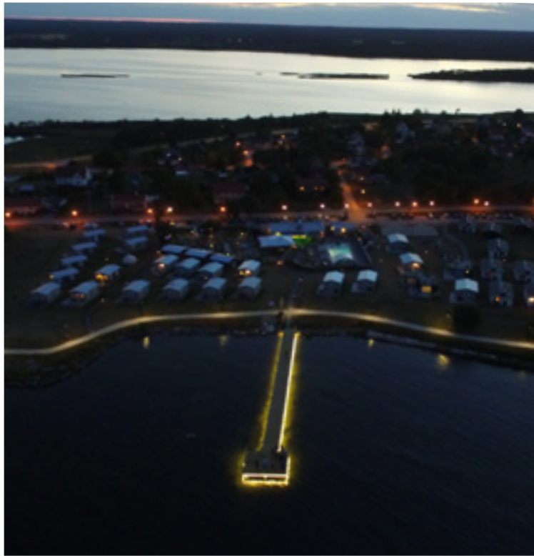
The pictures show Slite Strandby on Gotland. The splendid pier is illuminated by a 125-metre LED strip, 11 w/m. The strip is held in place with the help of X-Tray cable trays.
