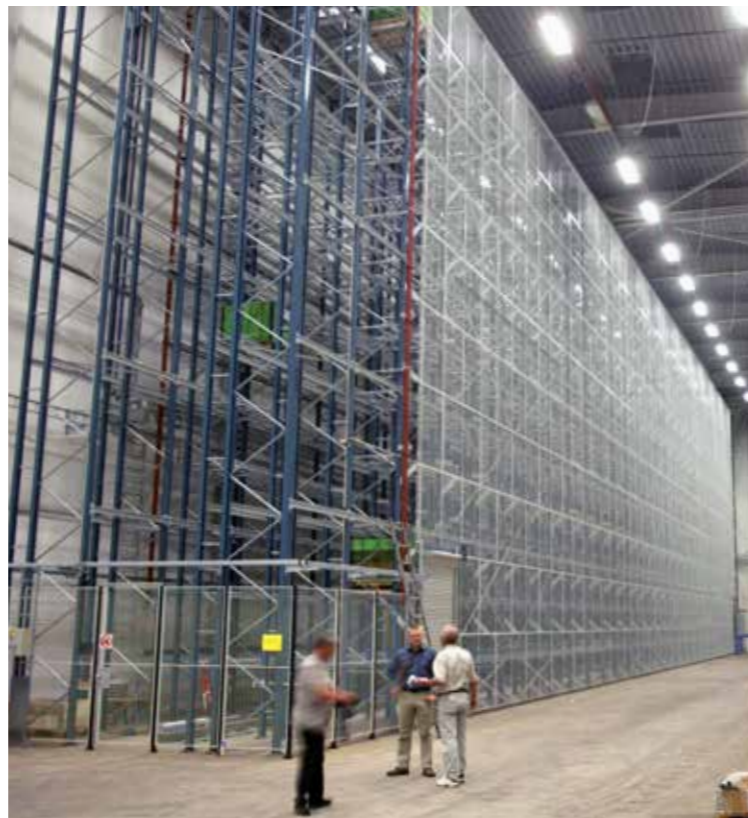
Axelent SafeStore with 50x60 mesh spacing. Project delivered to Scania in Oskarshamn.
